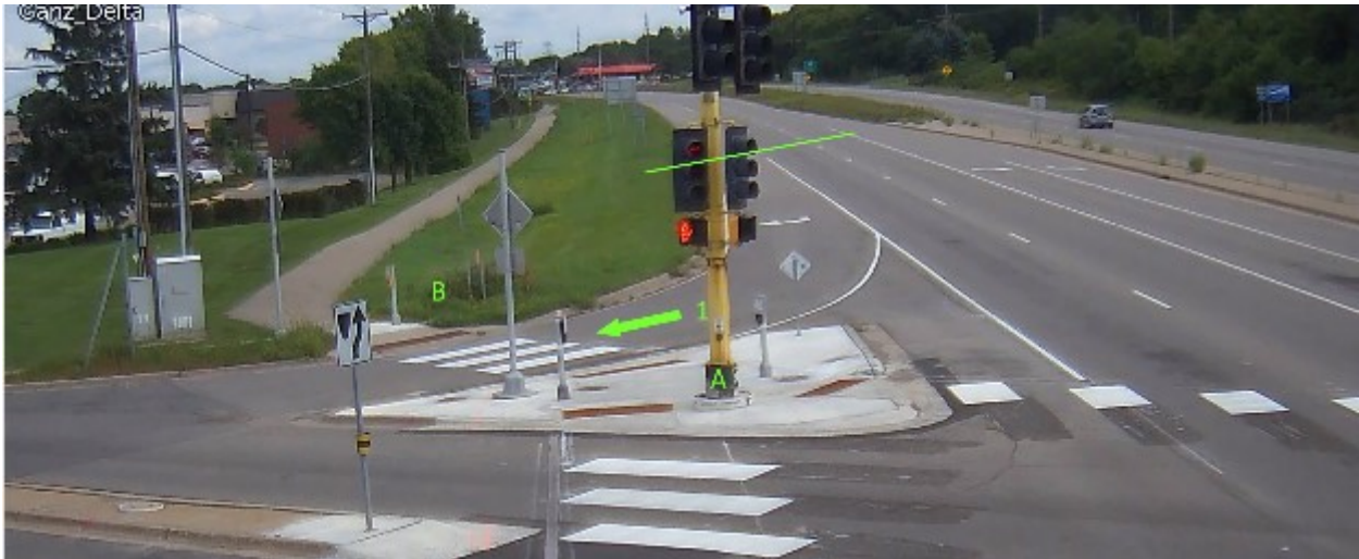
Figure 4-9 Site 1b in Burnsville at the northeast corner of TH-13 & Co Rd 11 AFTER the installation of a flashing LED sign.
