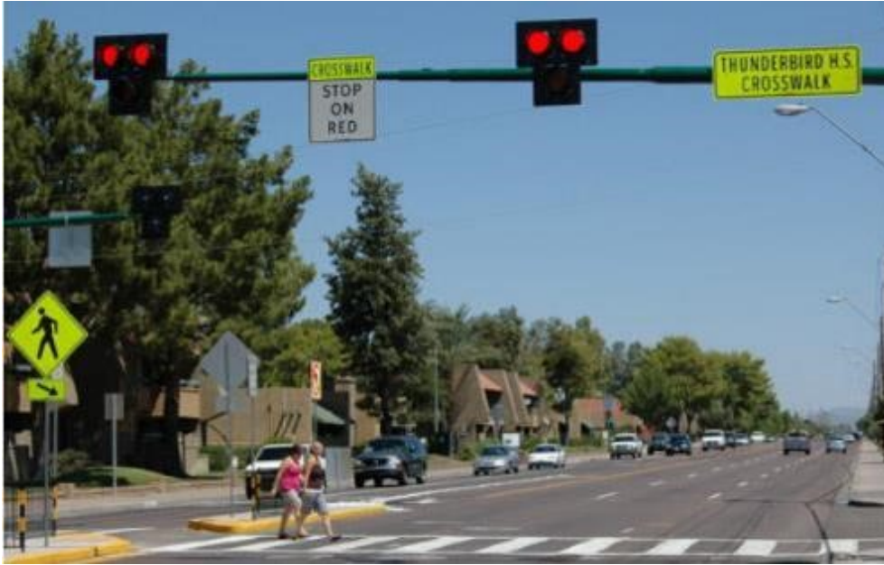
Figure 2-1 Example of Pedestrian Hybrid Beacon (PHB)
