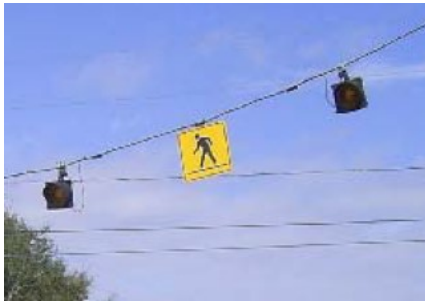
Figure 2-6 Standard overhead yellow flashing beacon
