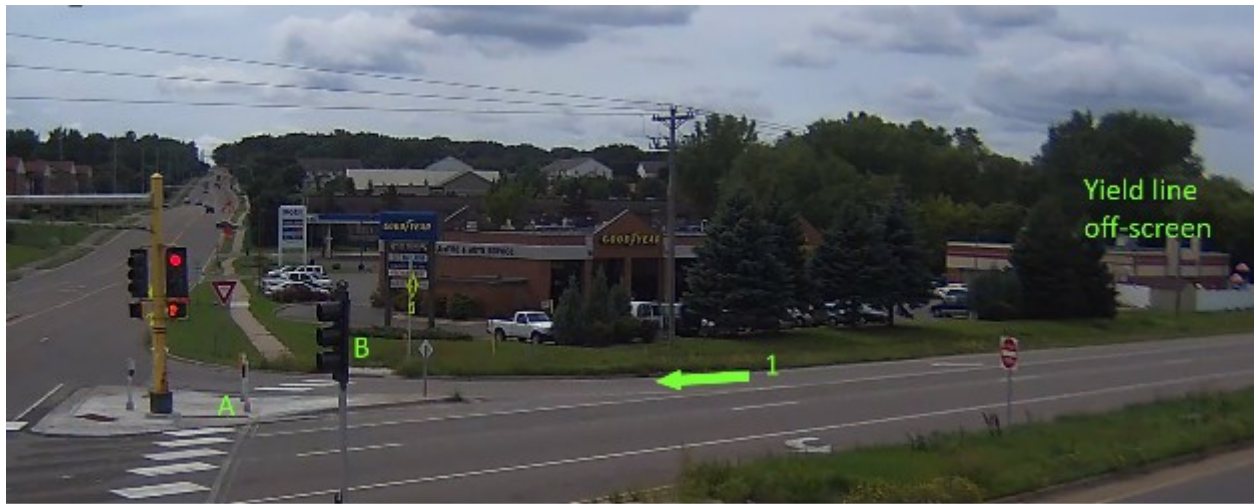
Figure 4-7 Site 1a in Burnsville at the southwest corner of TH-13 & Co Rd 11 AFTER the installation of a flashing LED sign.
