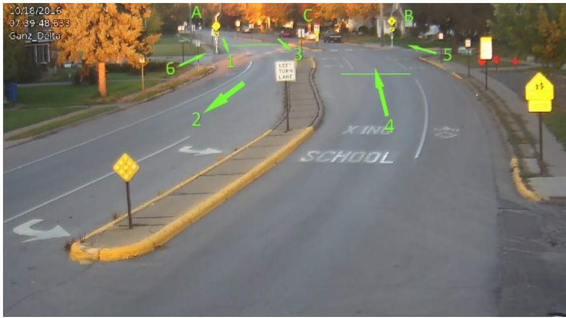
Figure 4-56 Site U4 in Winona at CSAH 32 & S Baker St.
