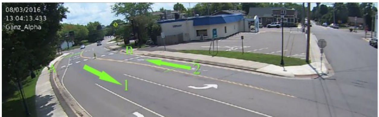
Figure 4-2 Site 7 in Maple Plain at TH-12 & Budd Ave.
