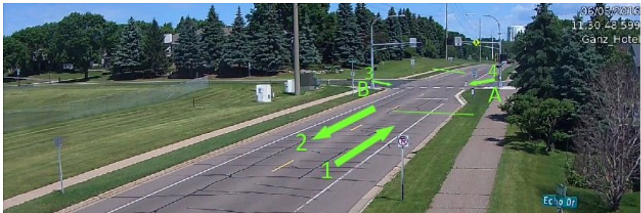
Figure 4-1 Site 6 in Burnsville at Co Rd 11 & 140th St.
