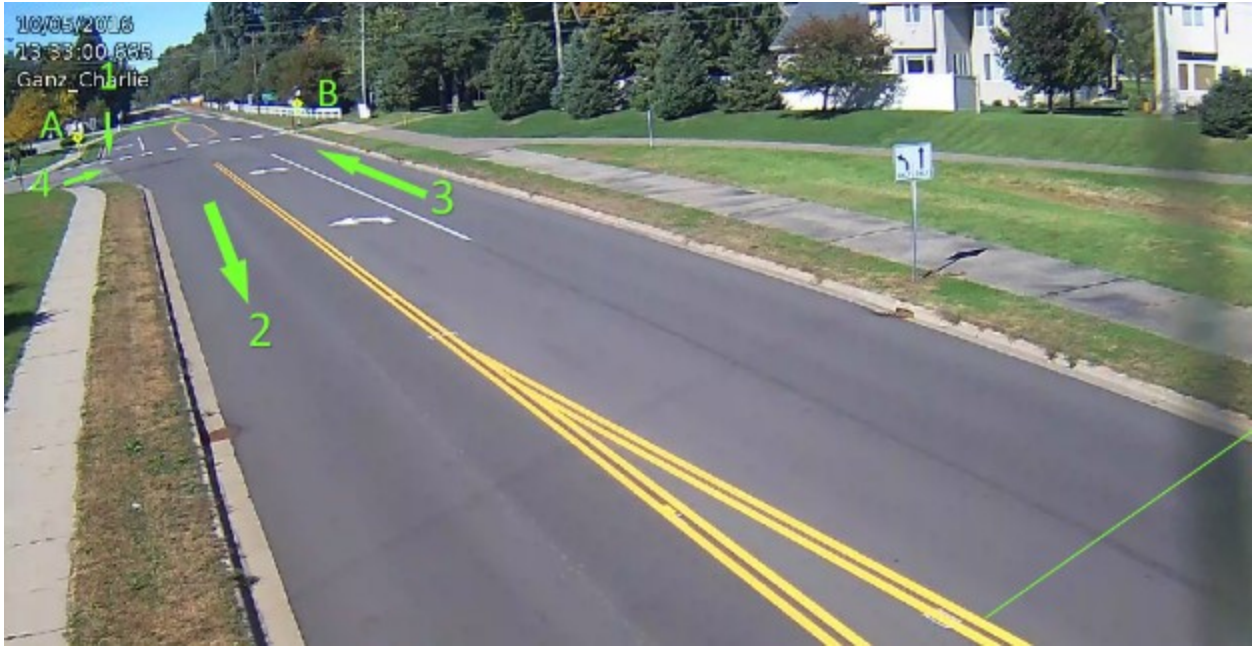
Figure 4-24 Site 20 in Champlain at W River Rd & 109th Ave N.
