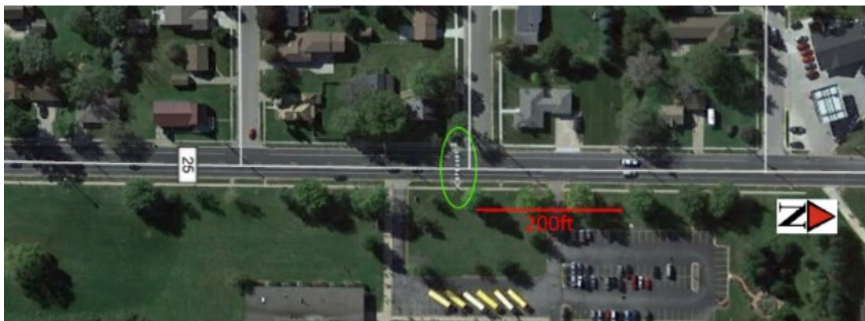
Figure 4-43 Aerial view of Site 41. Advanced warning sign icons correspond to the sign locations. The crossing is highlighted by the green oval.
